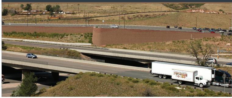
The design used a multipiece system to mimic area rock outcroppings. Four custom colors were used in the wall to show a sweeping motion near the top, which blends seamlessly with the surrounding scenery.
