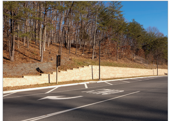
The finished wall is an important and attractive component in the widened road.
