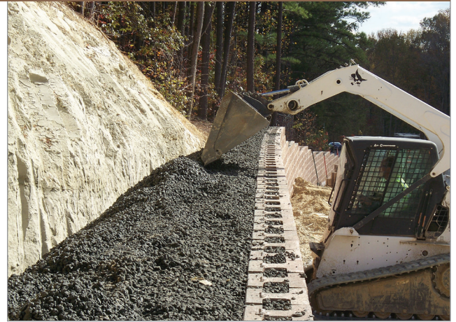
The Anchorplex™ retaining wall system can be used to build in areas too small for extensive excavation.
