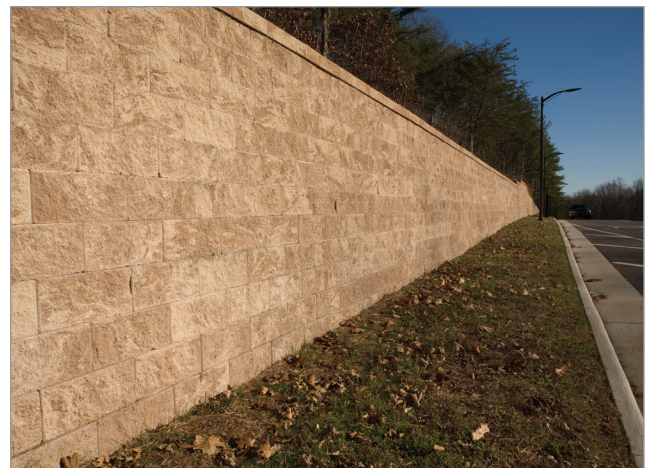
The Anchorplex™ retaining wall system built with Vertica® products made it possible for the road to remain open during most of the construction.
